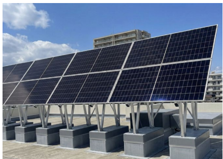
Flat roof installation example (with mounting frame)
