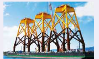
Jacket-type foundation to support offshore wind turbines
