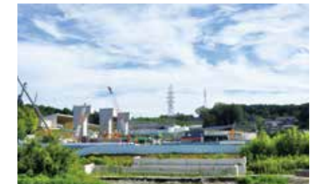
Construction site for the Gifu-ken Station on the Linear Chuo Shinkansen
