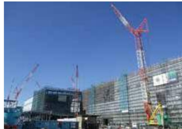
Construction site of a next-generation hot strip mill at Nagoya Works
