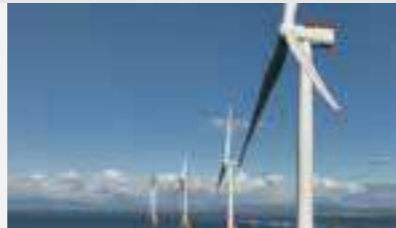
Japan's first jacket type foundation (Ishikari Bay offshore wind power plant), supporting an 8MW wind turbine
