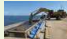
Construction using a soil modifier made from steelmaking slag
