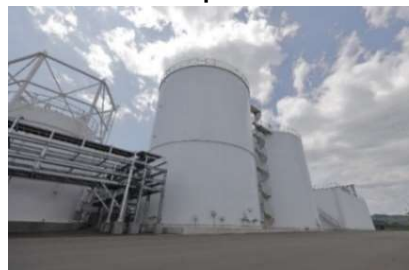
May 2023 Methane fermentation facility begins operation
