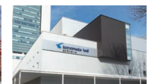
Kanamoto Hall (Sapporo Civic Hall) Housing a Large 1,500-person Event Hall as well as Small, Medium and Large Conference Rooms
