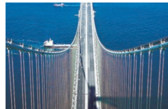
Improved construction efficiency for civil engineering Wire rods for high-strength suspension bridge cables
