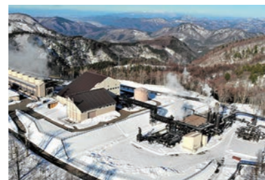
Wasabizawa geothermal power plant, one of the largest geothermal power plants in Japan, located in Akita Prefecture The eleventh in Japan is currently under construction.
