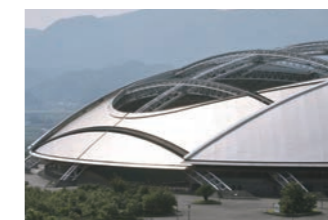
Prolonged service life and enhanced durability and reliability for the construction industry Titanium roofing
