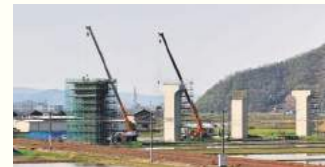
北陸新幹線の高架工事 Construction of an Elevated Structure for the Hokuriku Shinkansen
